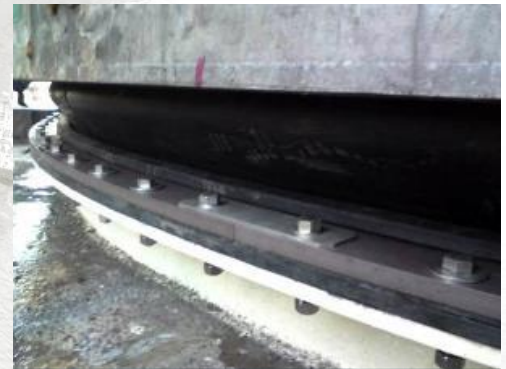
Cargo dome seal renewal
