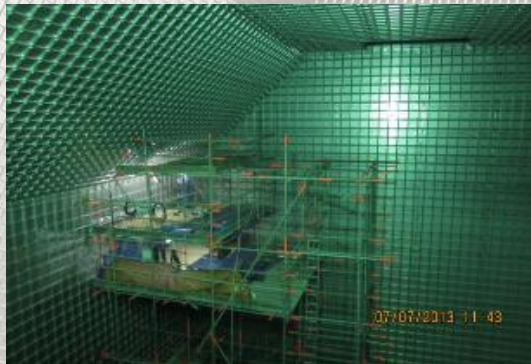
Top Chamfer Inspection
