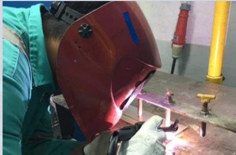
Invar welding training for welder
