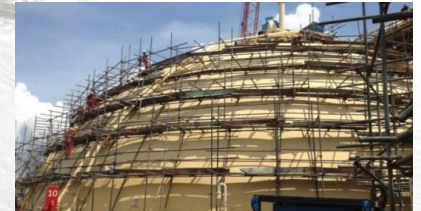
Full dome's staging work
