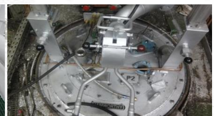
New Boiler Burner System Installation
