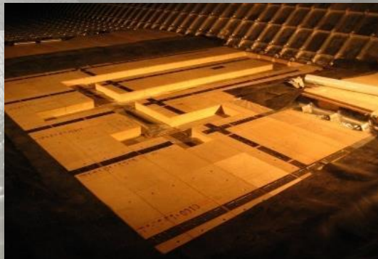
Secondary Barrier Repair
