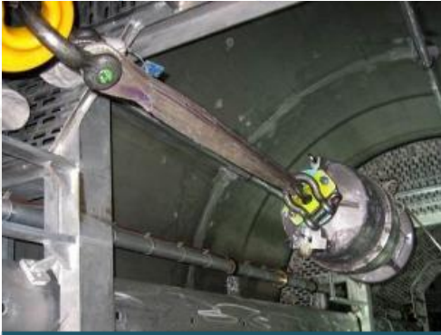
Cargo pump removal & overhauling
