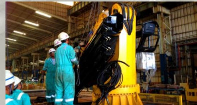
Installation of New Manifold Crane
