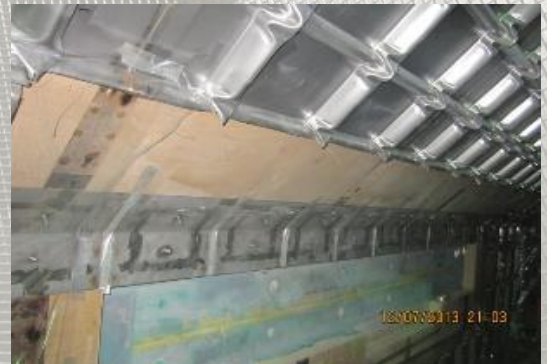
Secondary Barrier Repair
