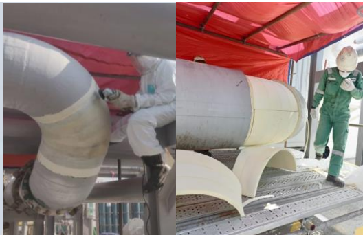
Cargo Cold Pipe Insulation Repair
