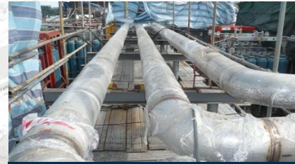
Installation of New Cargo Line
