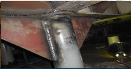
Fabrication Mooring Fairlead Foundation
