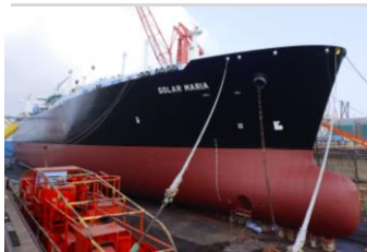
Type of works : Special Survey and BWTS Installation Year : June 2021
