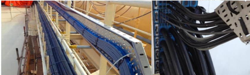
Power & Instrument Cable Renewal
