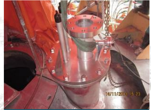
New CTMS / Penetration Installation
