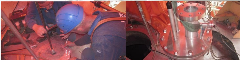
Cargo Tank Radar Gauging System Upgrading
