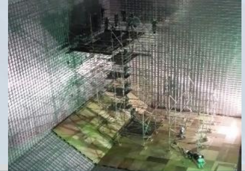
Scaffolding for LNG Cargo Tank
