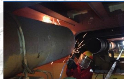
Ballast Line Renewal
