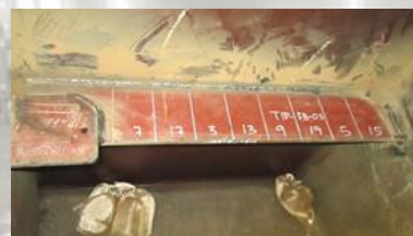
Fit and Weld Process
