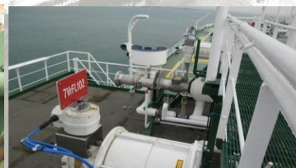
Installation of New Offloading Platform
