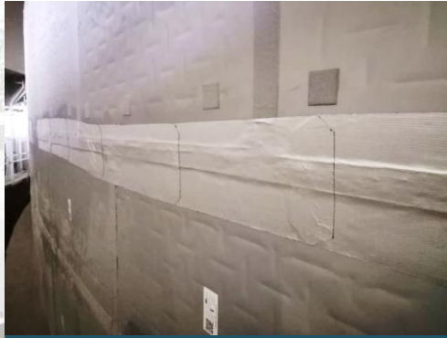
Insulation Repair
