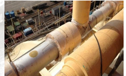
Cargo Pipe Insulation Renewal
