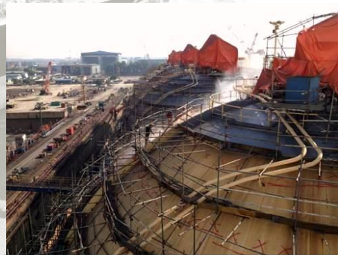
Full dome's staging & dome cosmetic work
