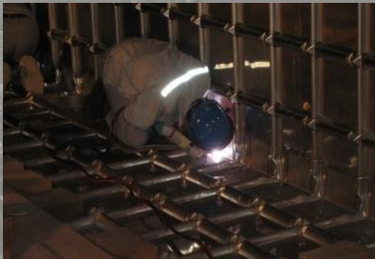
Mark III Membrane Welding
